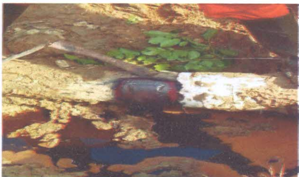
WORK DONE BY NAOC REPAIR TEAM (POINT A)
