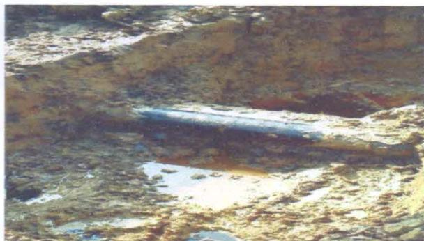
SPILL POINT AFTER EXCAVATION (POINT B)
