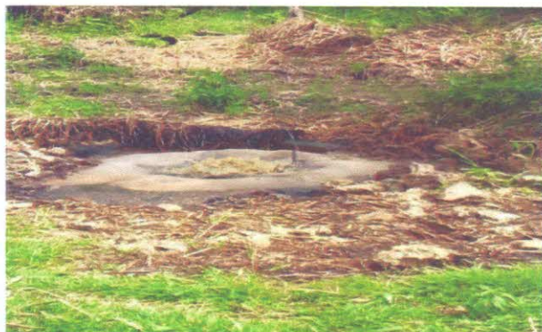
SPILL POINT BEFORE EXCAVATION (POINT B)
